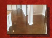
Polished Concrete (This floor has been dyed red during the polishing process.)
