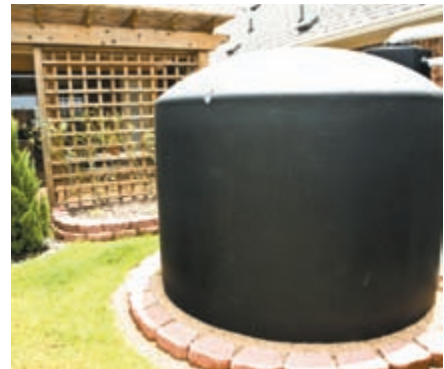
The Pouliots' two 1,750-gallon tanks harvest rainwater runoff for future use.
